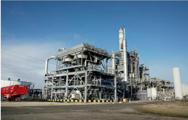
Figure 21: BOC's steam methane reforming facility in Teesside (Teesside Gazette)
